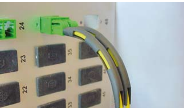
90° boot in horizontally mounted duplex adapters
